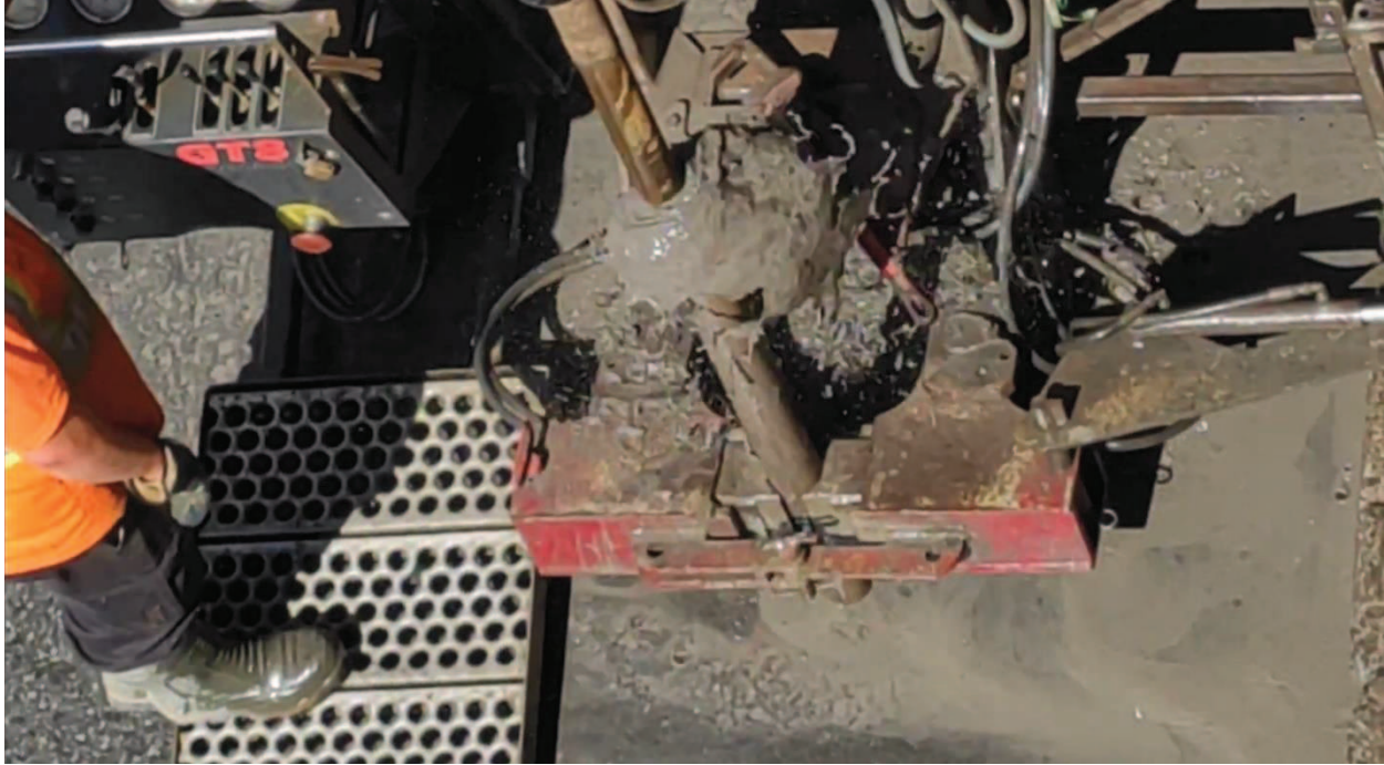
Picture 3 Drilling on Richelieu, corner Sainte-Marguerite. Video frame, taken August 5, 2020 2.56 PM
