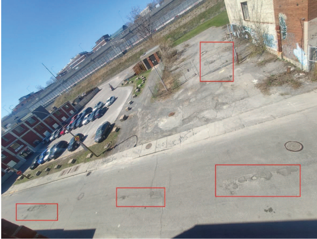
Picture 1 Some marks of drilled spots. Photo taken: April 13, 2021
