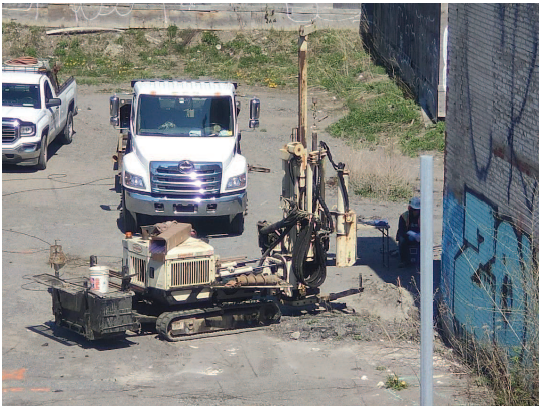
Picture 2 Drill machinery and trucks. Photo taken: May 7 2020 10.51 AM
