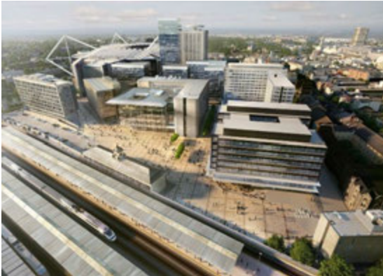
Cardiff's City Centre, Cardiff, Royaume-Uni Station de train et terminus d'autobus
